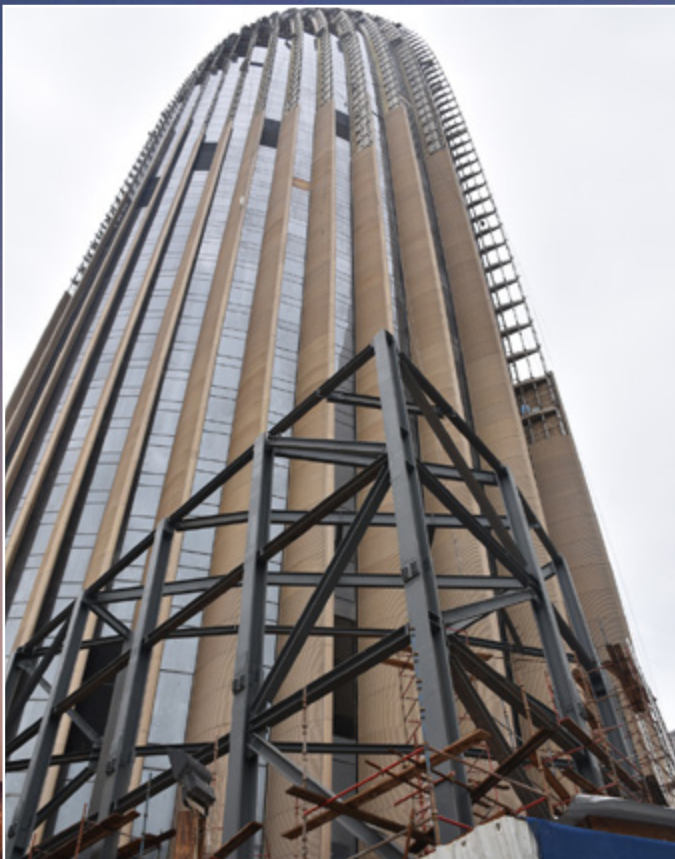
Secondary Steel Works for Façade
